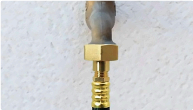
2. Connected and ready for the compressor.
